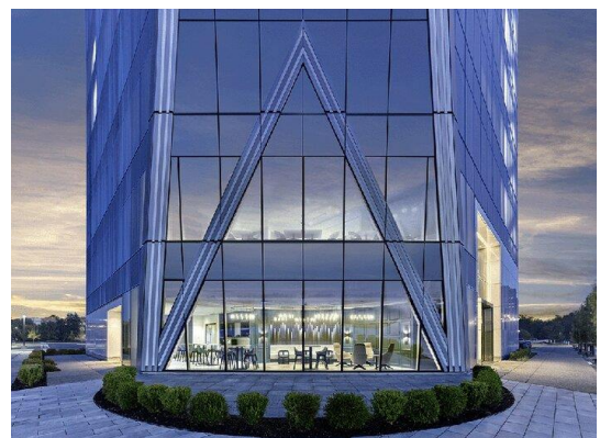
Morris James has moved its headquarters to a mixed-use campus on Avenue North Boulevard in Wilmington, Delaware. The new office — which is in north Wilmington rather than downtown, like the firm's former headquarters — has upgraded features and more conference room space. (Courtesy Photo)
